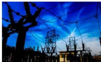
PLN Substations in Jakarta, Indonesia
